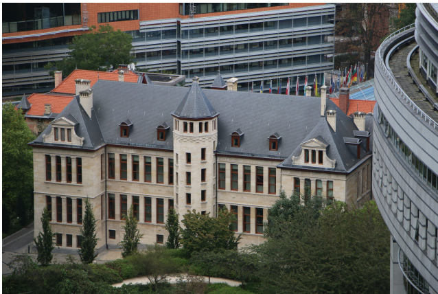
Premises: The main building of the Bavarian Representation in Brussels.
